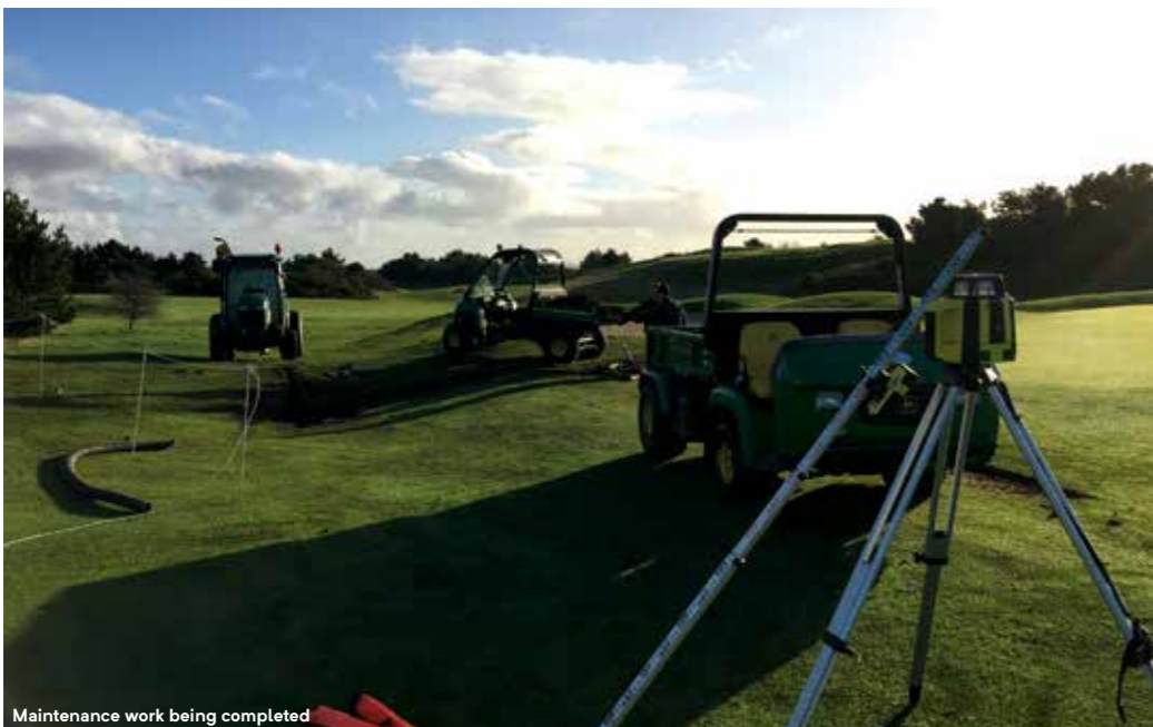
Maintenance work being completed
