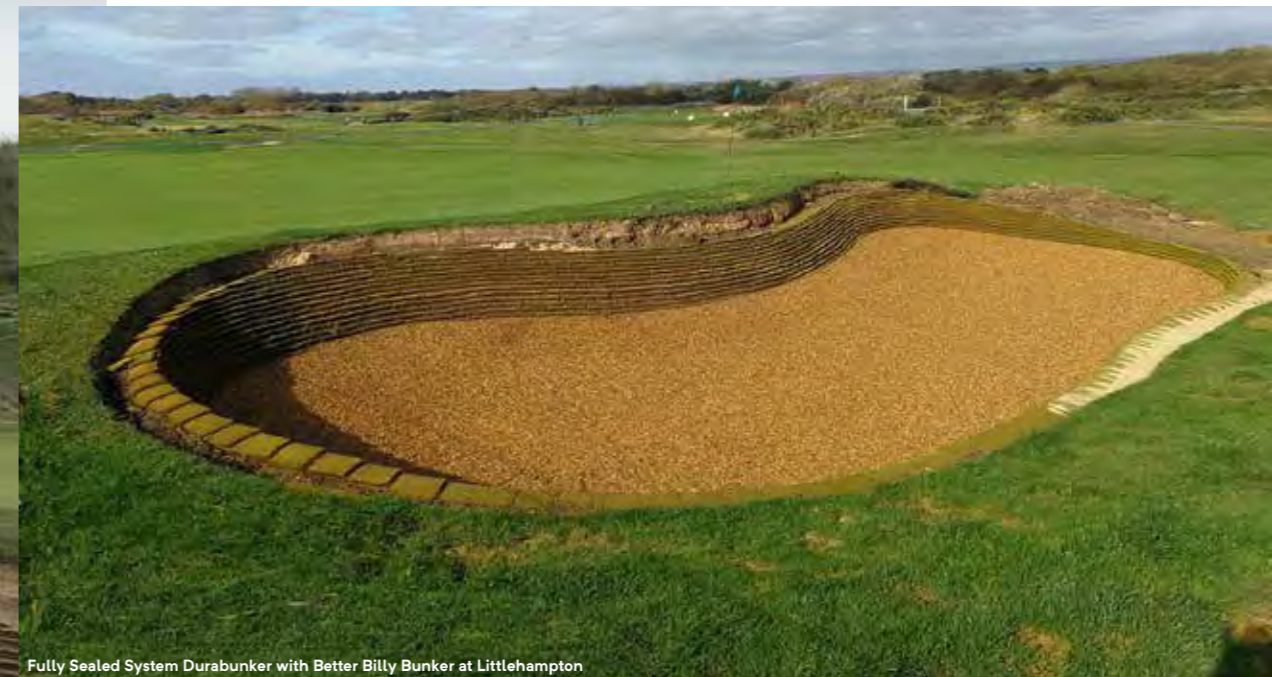
Fully Sealed System Durabunker with Better Billy Bunker at Littlehampton
