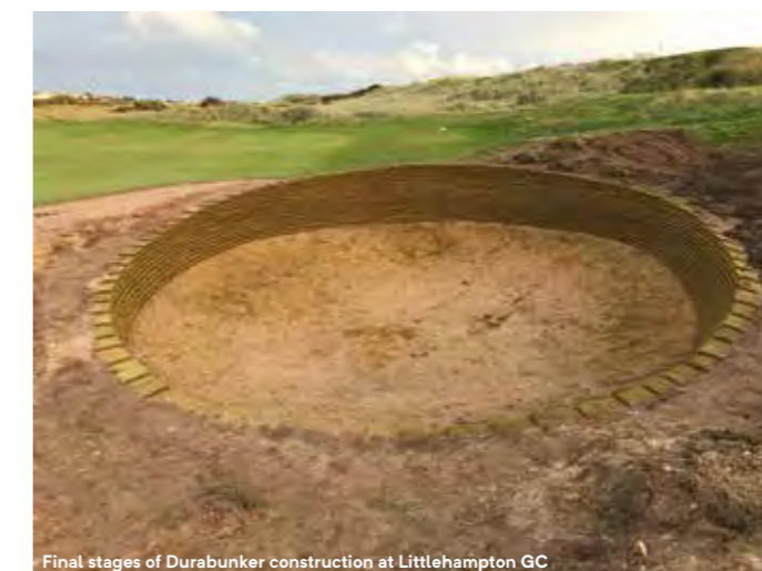
Final stages of Durabunker construction at Littlehampton GC
